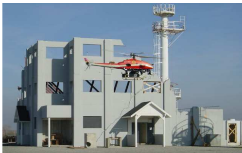
Fig. 2. The DART Collapsed Structure Rescue Training Site located in Mountain View, CA.
