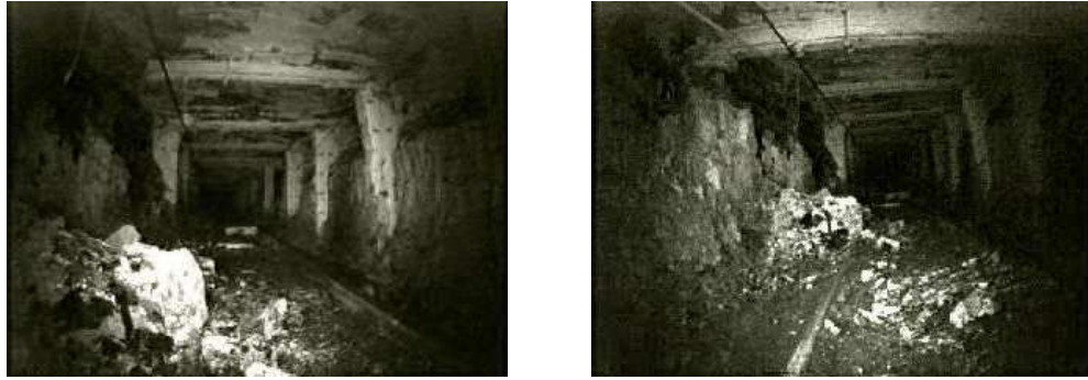
Figure 11: Camera images recorded while autonomously exploring the Mathies mine. Both image shows signs of degradation characteristic of abandoned mines, enabling mine safety personnel to assess the degree of deterioration.
